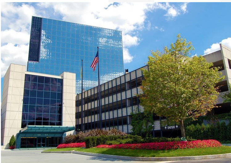
Front of Building and Parking Garage Entrance
